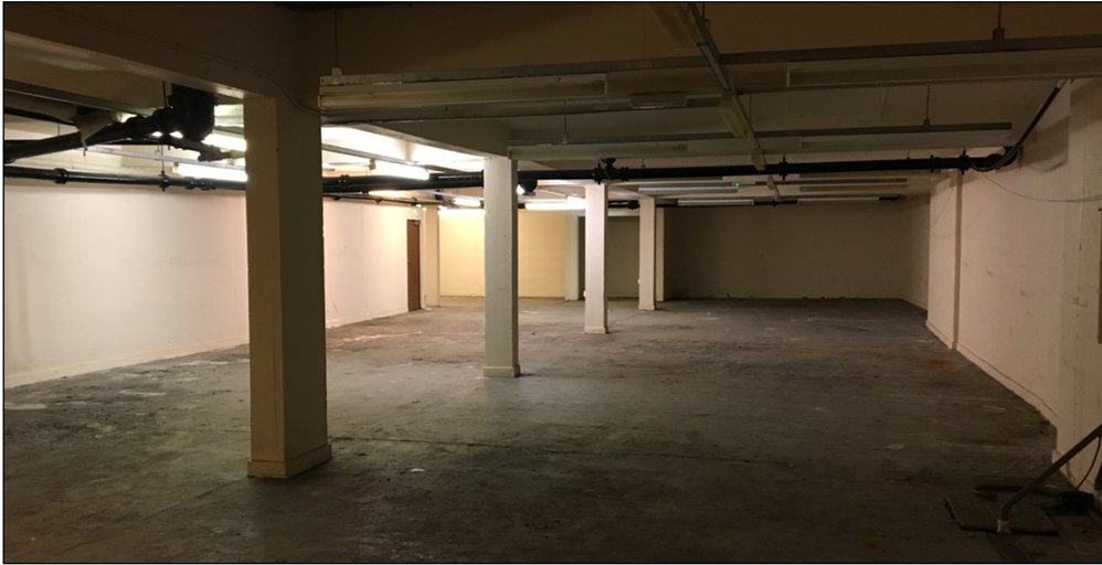
Image 5: Basement interior view
