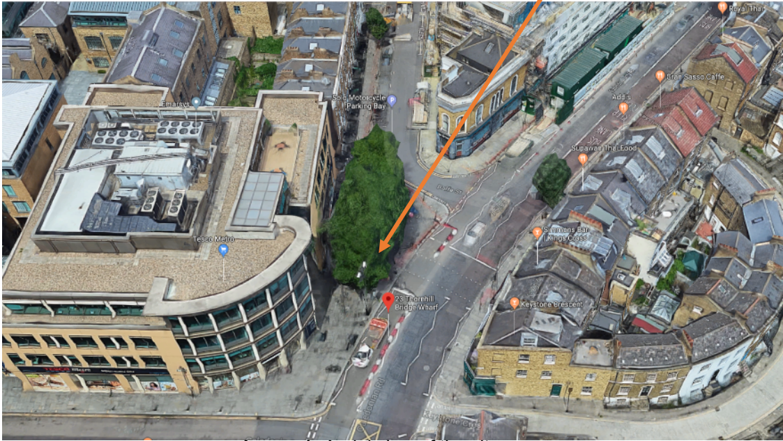
Image 1: Aerial view of the site
