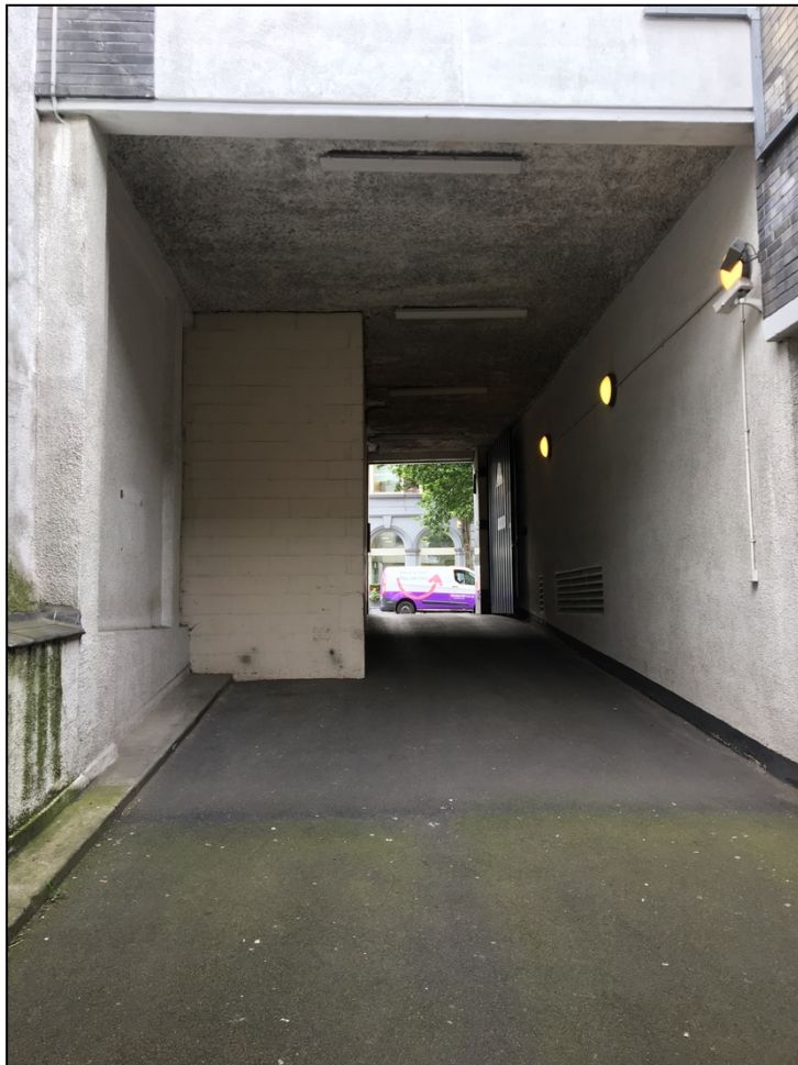
Image 5: Basement ramp facing upward towards St John Street
