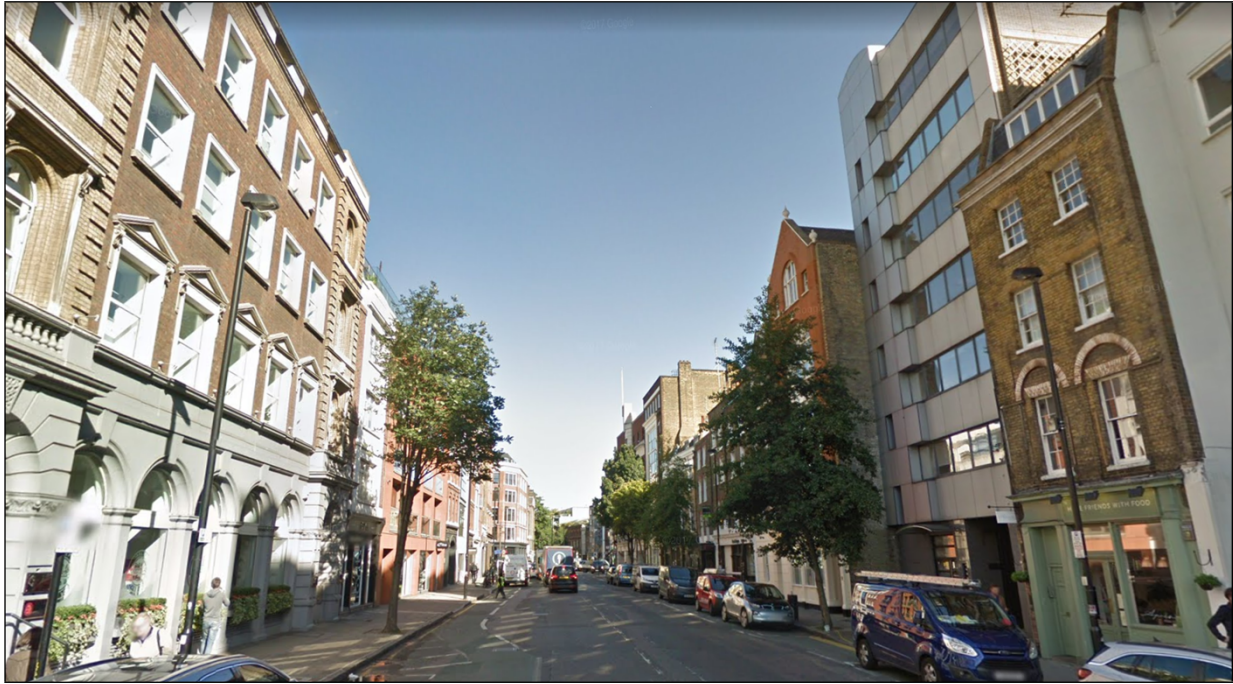
Image 3: St John Street, looking north. Site is shown on the right.
